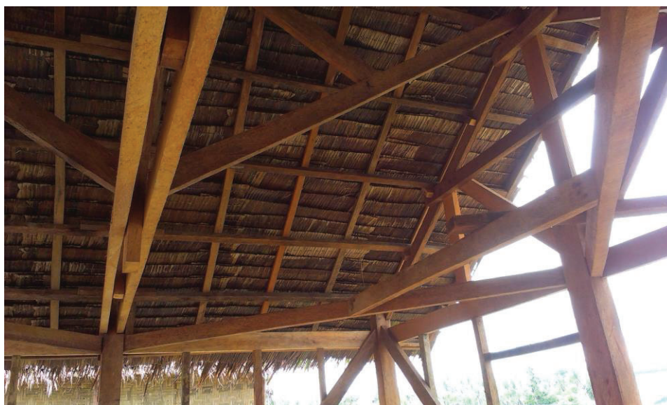
Figure 4: Roof structure (coco lumber) and nipa roofing. The nipa shingles are overlapped by 3". Project: Temporary shelters by IOM, All Hands Volunteers & Operation Blessing, Tagpuro, Leyte, Philippines. (Photo R. Dodds, Humanitarian Shelter Working Group)
