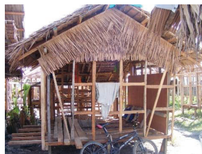
Figure 2: A shelter with coco lumber framing and nipa roofing in Tanauan, Tacloban, Philippines by NGO Green Mindanao. (Photo: K. Balson, Building Research Establishment Ltd.)
