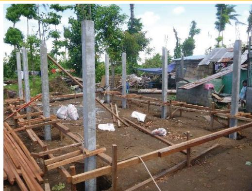
Figure 2: Reinforced concrete columns have been erected for this core shelter in Tabontabon, Leyte. Credit: Philippines Red Cross Haiyan Shelter Programme (Photo W. Eastwood)
