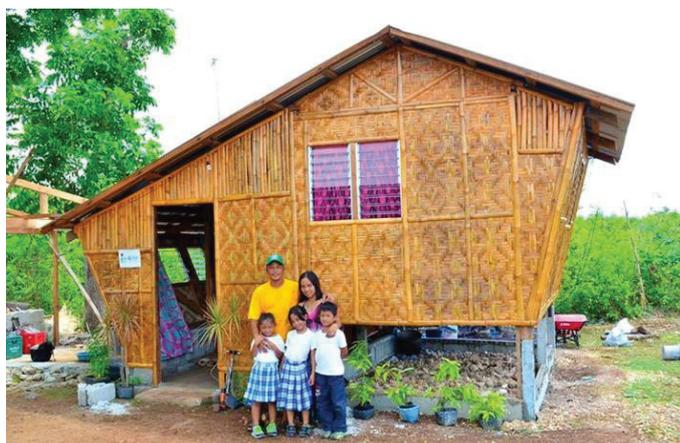
Figure 3: Shelter with amakan wall cladding, YPDR PAH Joint Housing Program, Bantayan Island, Philippines. (Photo: Joseph Ferris III, YPDR)
