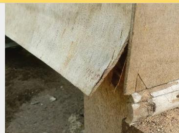
Figure 2: warping of untreated plywood, Bantayan Island, Philippines. (Photo: R. Dodds, Humanitarian Shelter Working Group Philippines 2014)
